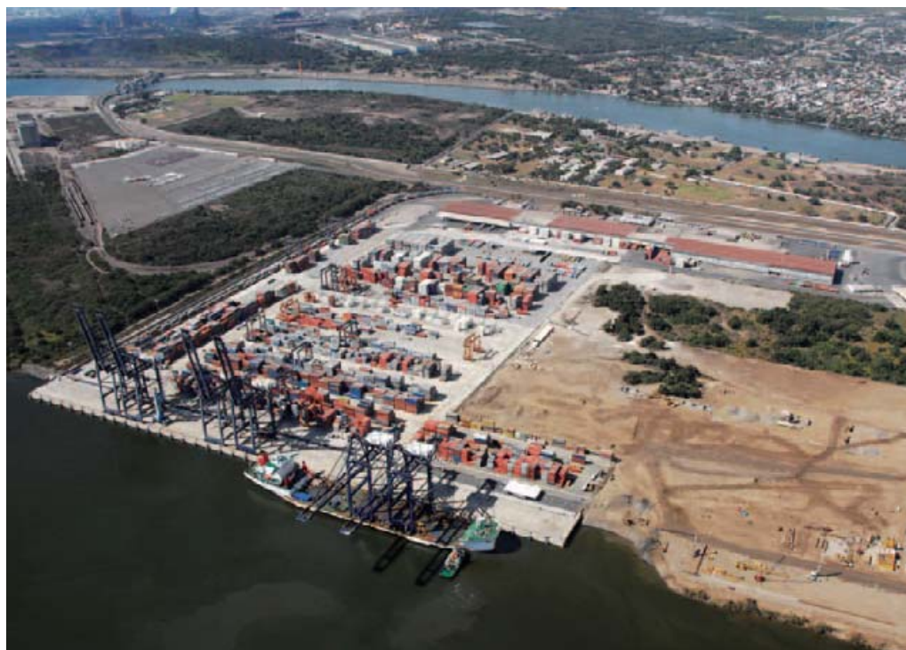
Mexico's L.C. Terminal Portuaria de Contenedores, situated in the highly industrial deep-water port of Lázaro Cárdenas.
